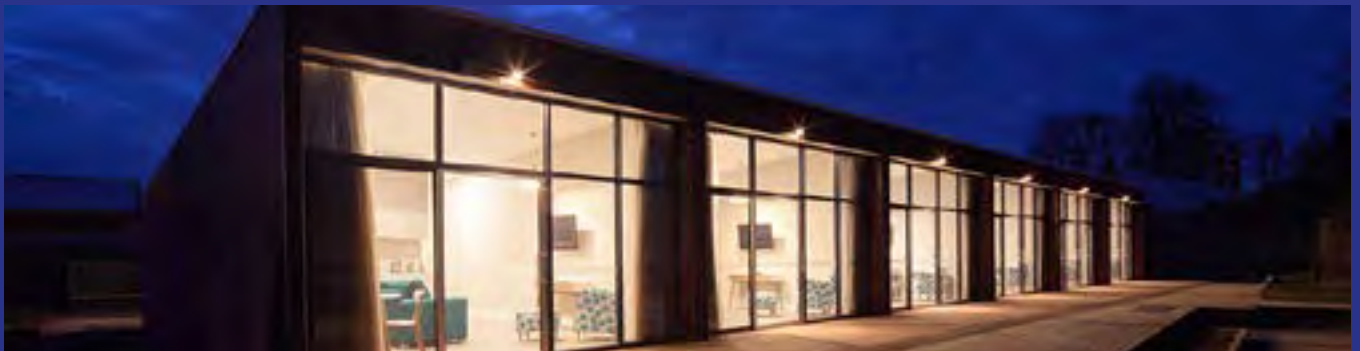
Project: Ballarat Health Services Cancer Accommodation Units, Lake Wendouree Services: Modular Design - 6 modular pre-fabricated health care units Client: Precom
